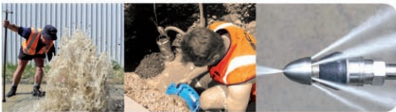
Pipe & Drain Repairs & Unblocking
