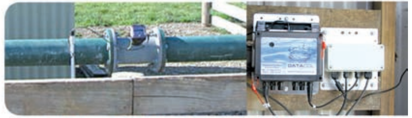
Irrigation Watermeter Installation
